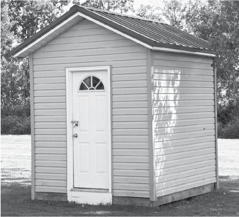
Courtesy photo Pictured is one of three buildings at Newman Park that received new roofs.
